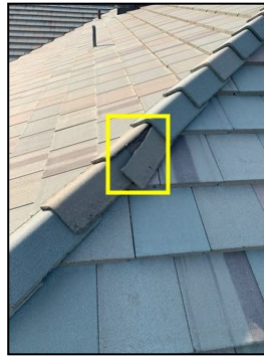
Broken ridge cap at north/east hip
