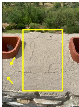
Moderate cracking of chimney cap – north
