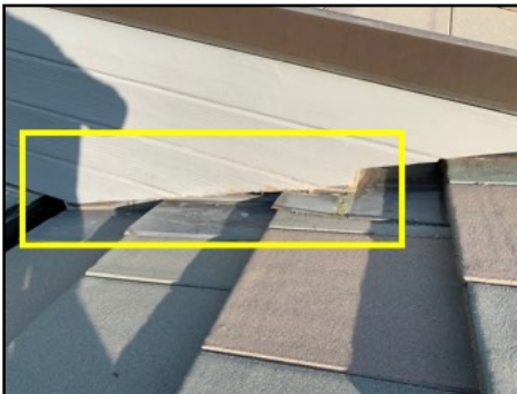
Wood cladding covering the exterior walls at south/west aspect has inadequate clearance from roof covering, showing signs of damage
