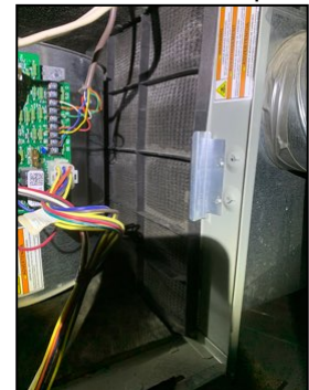
Crawlspace furnace filter at return air plenum, appeared clean
