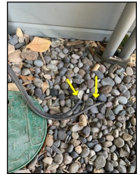
Abandoned electrical wiring at east aspect
