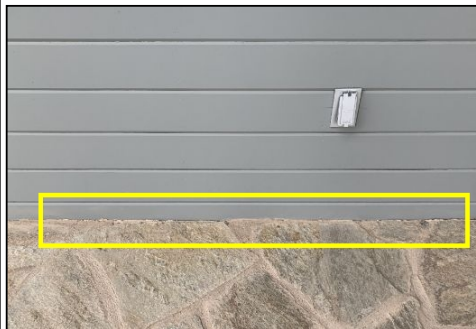
Inadequate clearing from grade at north patio
