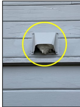
Clogged dryer vent at west
