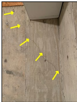
Ascending closure crack observed at north/east corner of projector room
