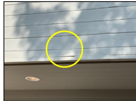
Loose wood cladding at south garage
