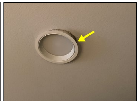
Loose light fixture above shower in bathroom #3
