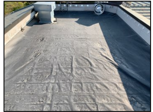
Rolled rubber roof covering
