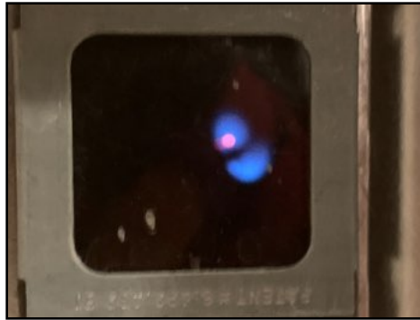
Water heater sealed burner compartment, pilot is lit
