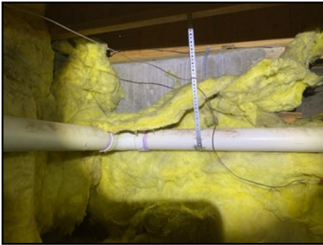
Loose insulation at north/east aspect
