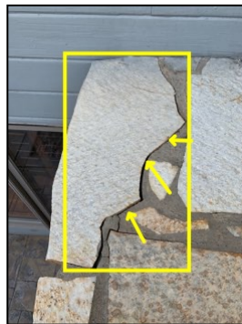
Loose stone at west retaining wall
