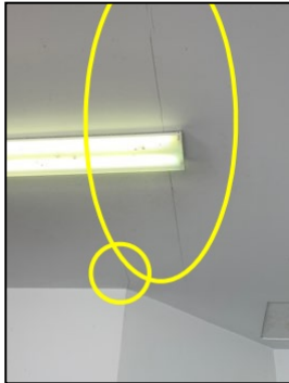
Unusual crack pattern at garage ceiling
