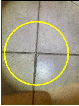
Cracked grout observed near garage service door
