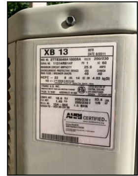
A/C condenser unit manufacturer data plate - North
