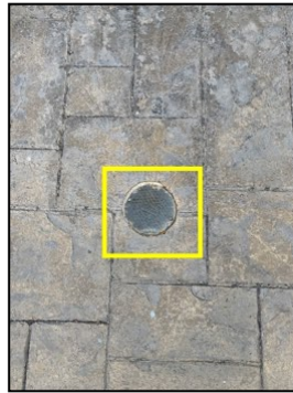
Waste drain clean-out at west
