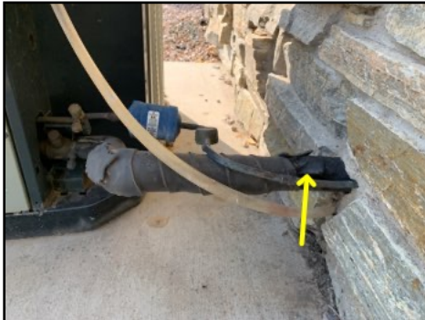
Insulation on A/C condenser unit refrigerant line for south unit is damaged
