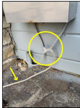
Exposed electrical wiring at north lower level
