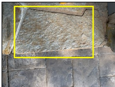
Loose stone observed at stoop to ADU unit
