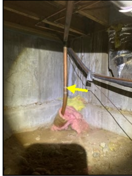
Main water service at south/east crawlspace
