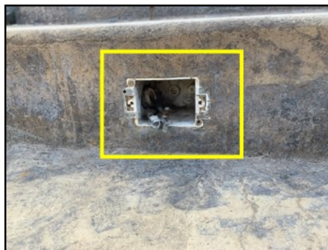
Exposed junction box at rear exterior stairwell
