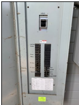
Main electrical service panel
