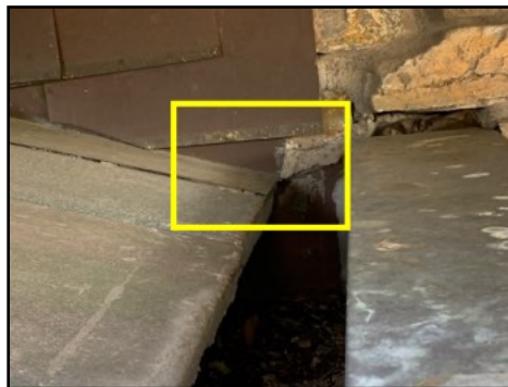
Kick - out flashing absent at south/east
