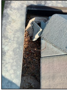
Dirt/debris observed in gutter at north/west aspect
