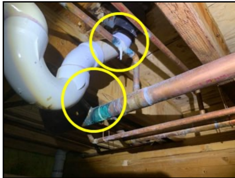
Heavy corrosion observed on water supply pipes in crawlspace beneath shower #1
