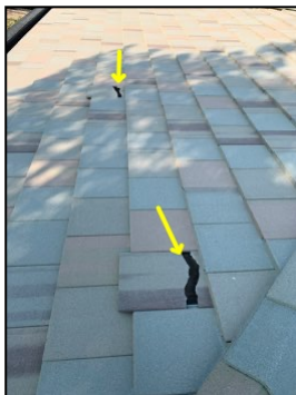
Cracked/broken tile at southern slope
