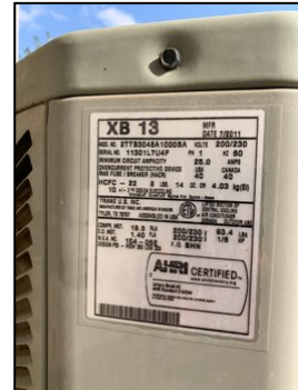
A/C condenser unit manufacturer data plate - South
