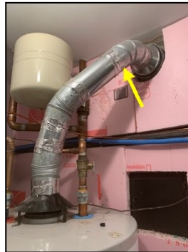
Water heater vent pipe exhausts into chimney flue
