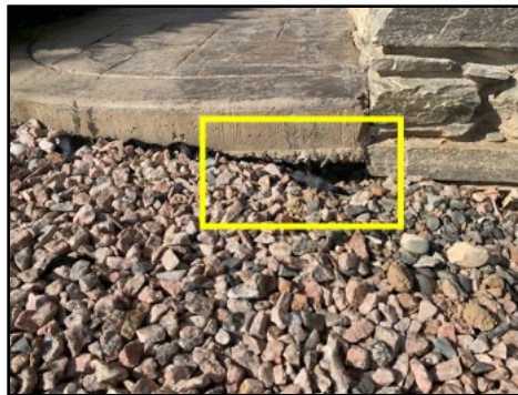
Undermining of soil beneath east aspect of front walkway
