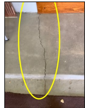
Crack observed at stoop in garage, signs of displacement
