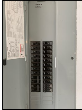
Power remote distribution panel in the garage
