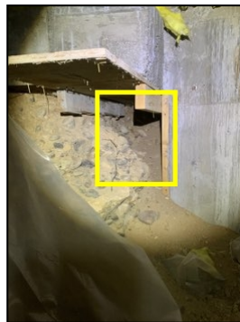
Loose soil beneath footing at south/west
