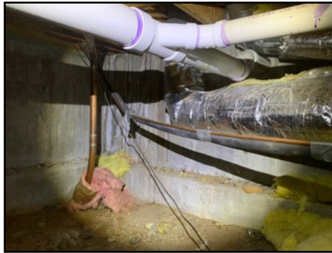
Loose/absent insulation at south/east
