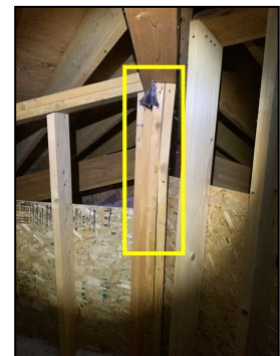
Inadequate support of hip rafter at south/west
