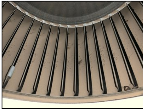
Furnace in mechanical room blower vanes, appear dirty
