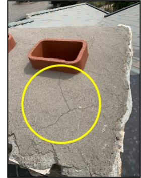
Moderate cracking of chimney cap-south
