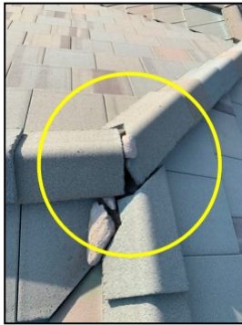
Ridge cap installed at south/west has left gaps exposing roof to moisture intrusion
