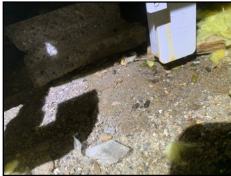
Rodent droppings beneath crawlspace furnace
