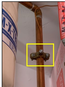
Water pipe bond at water heater supply
