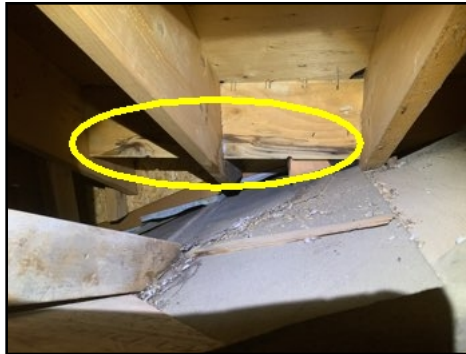
Dry moisture stains observed at south/east valley
