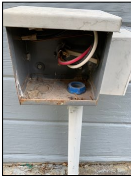
Abandoned electrical wiring at north/west aspect
