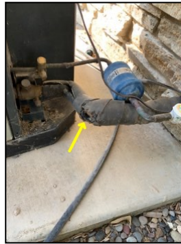
Insulation on A/C condenser unit refrigerant line at north is damaged
