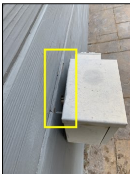
Junction box at west exterior is improperly fastened
