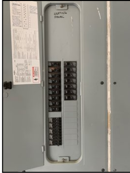
Lighting remote distribution panel in the garage
